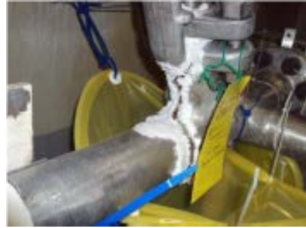
Boric acid leak in a nuclear plant.
